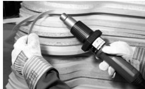
Shrinking cable sleeves
